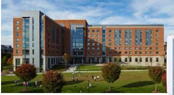
UMCP Frederick Hall, Maryland (USA)
